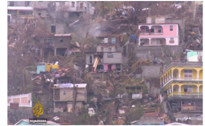
(a) Hurricane Maria turns Dominica into 'giant debris field' https://t.co/rAISiAhMUy by #AJEnglish via @c0nvey https://t.co/l4zeuW4gkc
